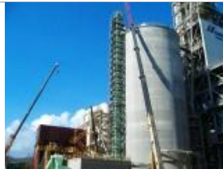
Scaffold (over 125ft)
